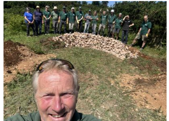
Photo: Ranger and volunteers constructing a reptile hibernaculum
